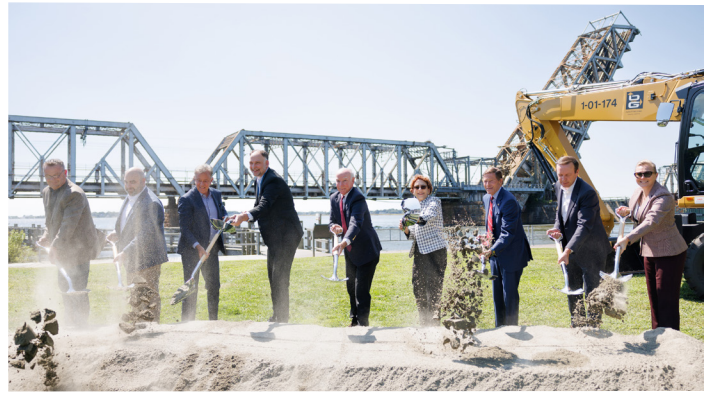
Alongside the State of Connecticut and the FRA, Amtrak broke ground on the new Connecticut River Bridge (between Old Saybrook and Old Lyme, Conn.) that will offer a 55% speed increase from the existing 1907 bridge.
