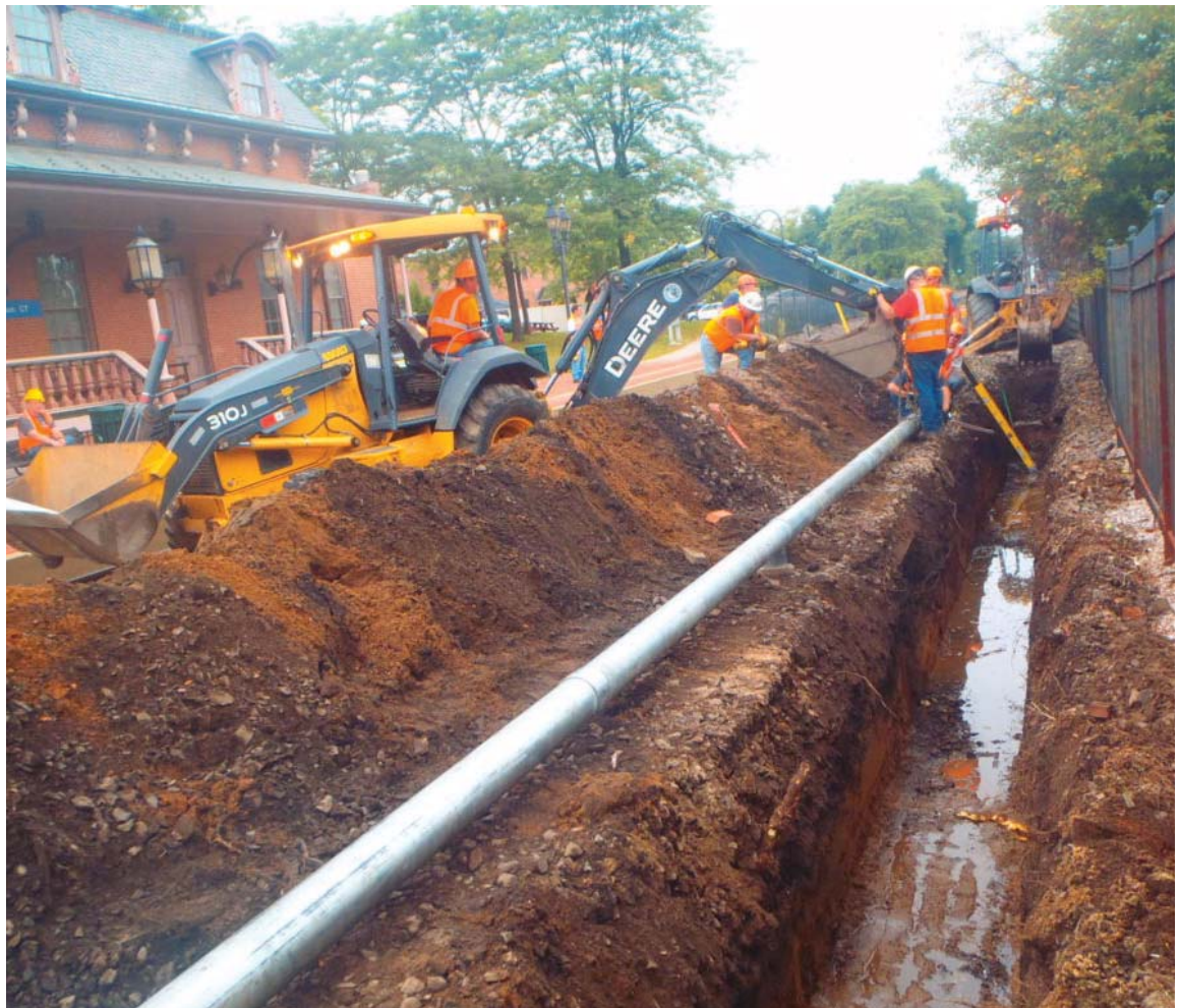
New Haven-Hartford-Springfield Rail Program: Construction of signal upgrades. Photo courtesy of Connecticut Department of Transportation.
